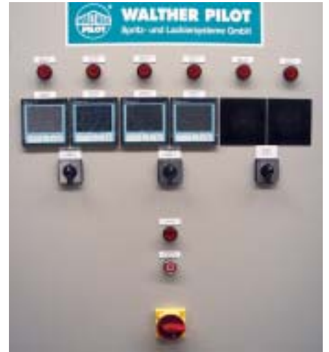
Control cabinet with meters for level monitoring
